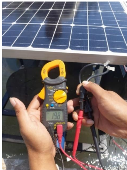
Gambar 4.9 Proses Pengambilan Data Panel Surya
