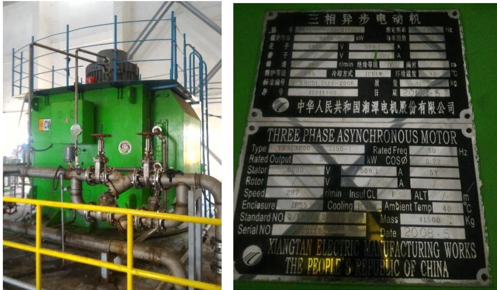
**Gambar 4.1** Motor *Circulating Water Pump* PLTU Paiton Unit 9
